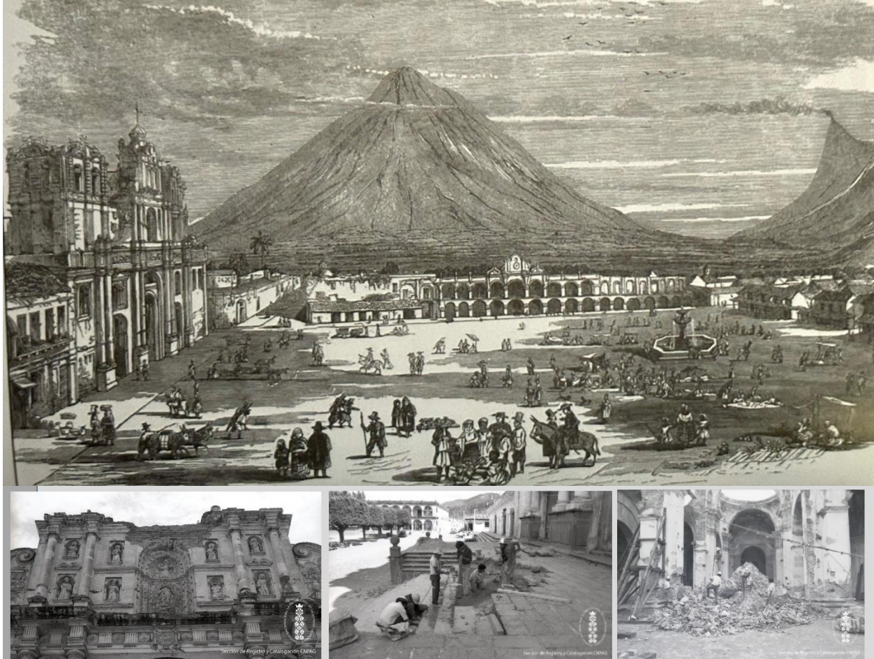
Figure 7: Top: An illustration of the Central Plaza published in The Illustrated London News on August 3, 1856 (Bell, 2010, p. 18). Note the bell tower to the north of the façade of the cathedral. Bottom Row: Photographs showing the collapse of the central portion of the cathedral façade, damage to the steps below, and within the ruins. (Photos courtesy of CNPAG Sección de Registro y Catalogación).
