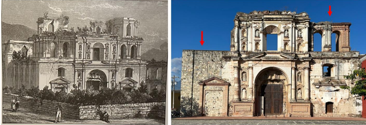
Figure 8: Left: Illustration of Compañía Jesús from The Illustrated London News , March 12, 1859. (Bell, 2010, p. 79). Right: Photograph of the façade of the church of Compañía Jesús in 2025. The red arrows point to portions of the structure that collapsed and have been reconstructed.
