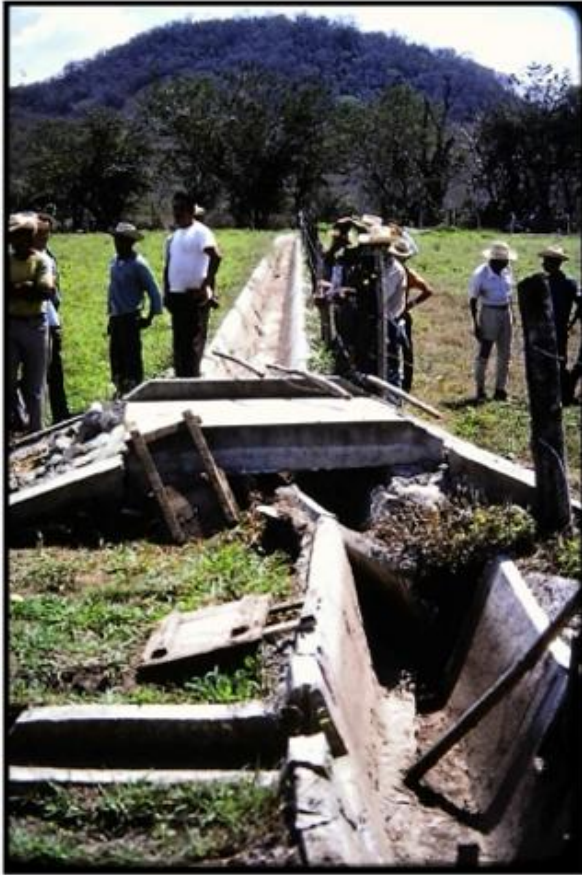
Figure 43: Photograph of the concrete irrigation canal offset by slip of 93 cm of the Motagua fault in Finca Los Limones east of Gualán. Left, February 1976; Right, July 2021.
