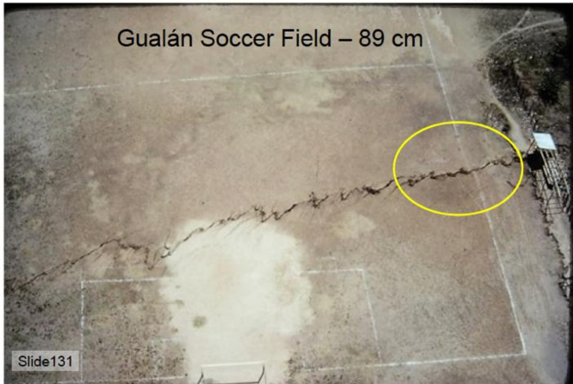
Figure 42: Oblique aerial photograph of the Gualán soccer field viewed northward showing the 1976 earthquake moletrack. A left-lateral offset of 89 cm was measured across the white sideline stripe (Plafker, 1977).
