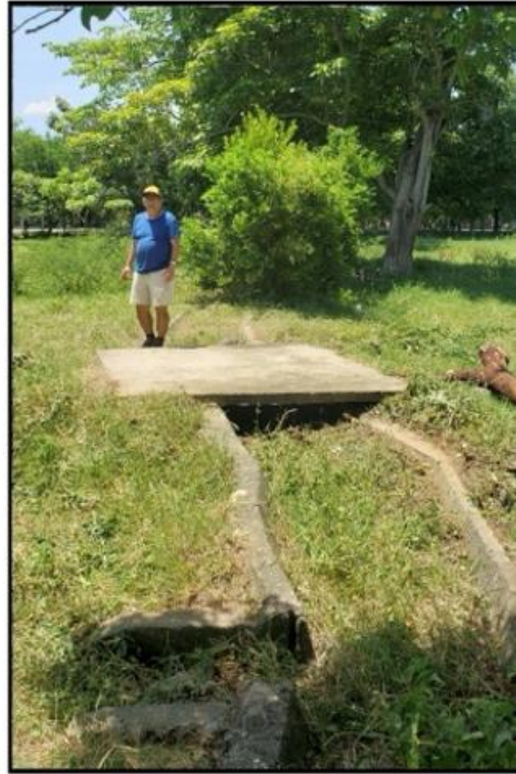
Figure 43: Photograph of the concrete irrigation canal offset by slip of 93 cm of the Motagua fault in Finca Los Limones east of Gualán. Left, February 1976; Right, July 2021.
