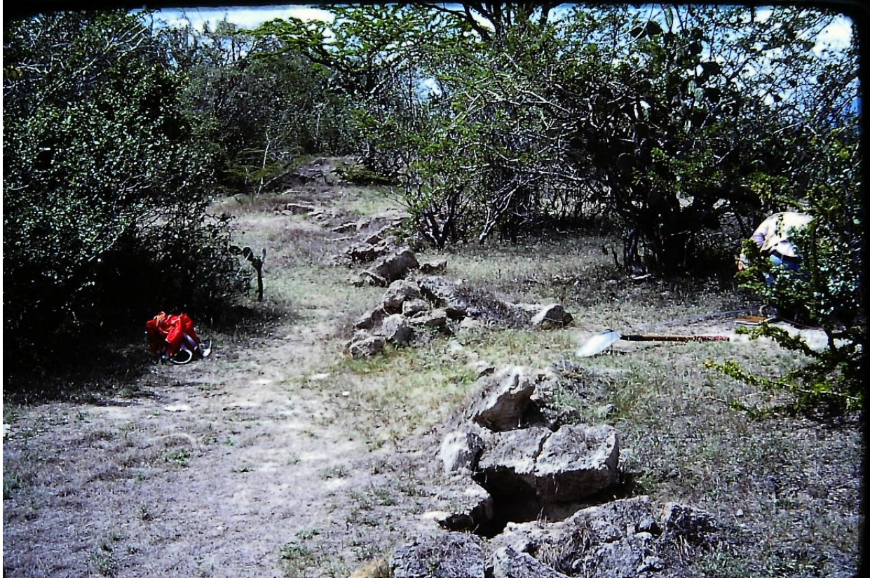
Figure 15: Installation of monitoring monuments across the mole track surface rupture for afterslip measurements. Plafker archive slide 1507
