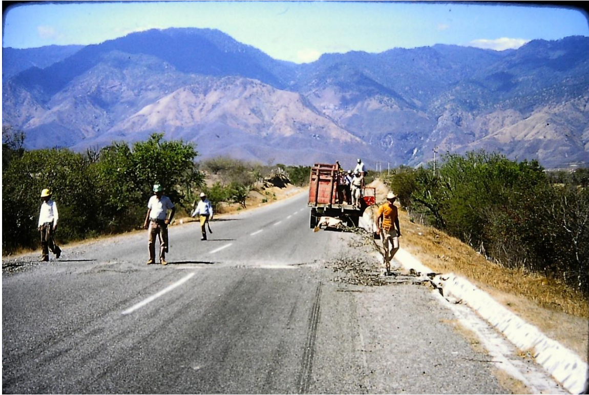
Figure 16: A total of 31 cm of left-lateral afterslip was recorded at the Estanzuela section 610 days after the earthquake (Bucknam et al., 1978).
