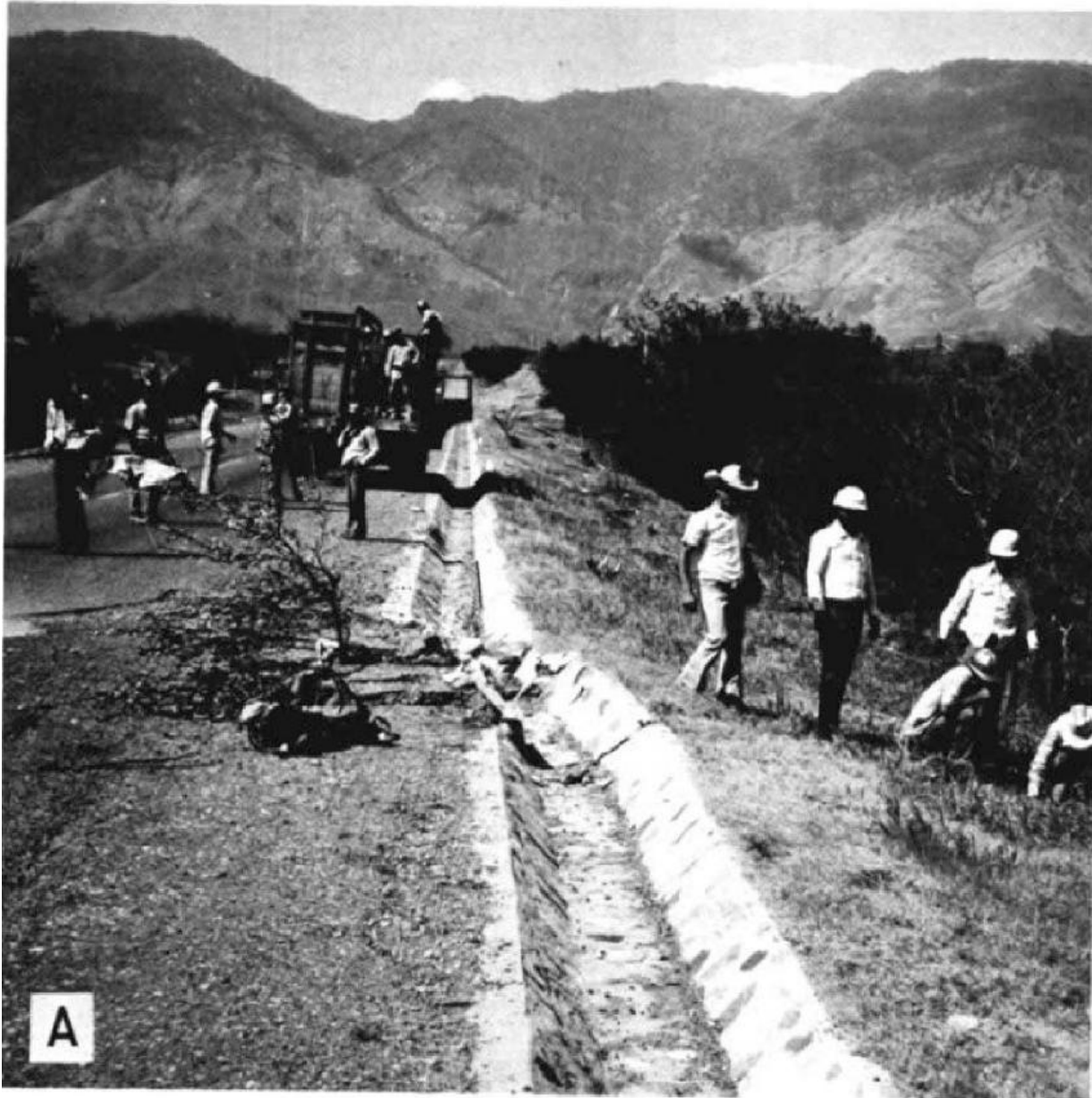
Figure 14: Offset Highway CA-10 north of Zacapa in February, 1976. From Bucknam et al. (1978).
