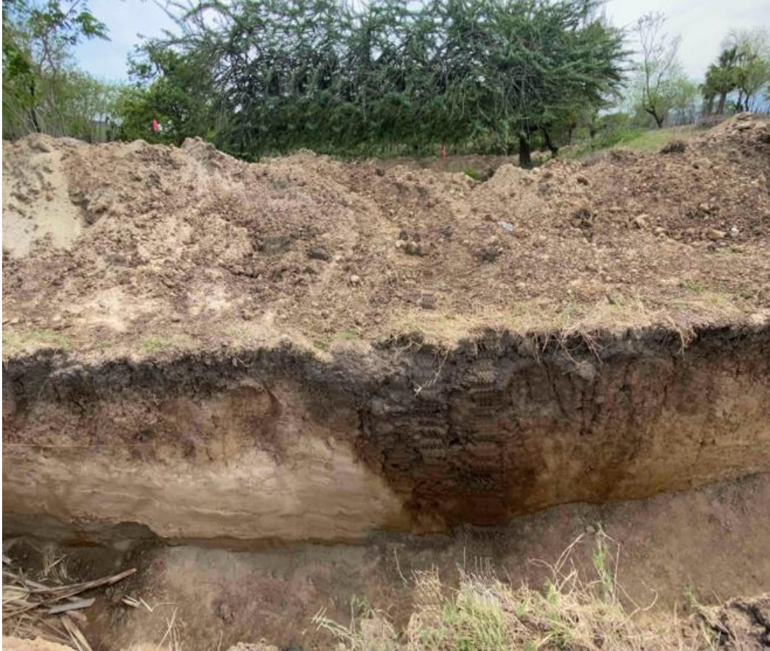
Figure 48: Photograph of the west wall of Trench 2 showing multiple, inset organic-rich fissures along the fault trace.
