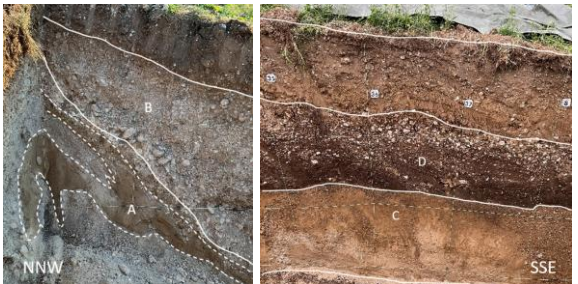
Figure 7: (a) Evidence of fault-related deformation: sands and gravels of the fluvioglacial units A and B with high angle (340/85) close to the northern scarp; (b) Evidence of seismic shaking: sand and gravels liquefactions (unit C) on the south part of the excavated wall.
