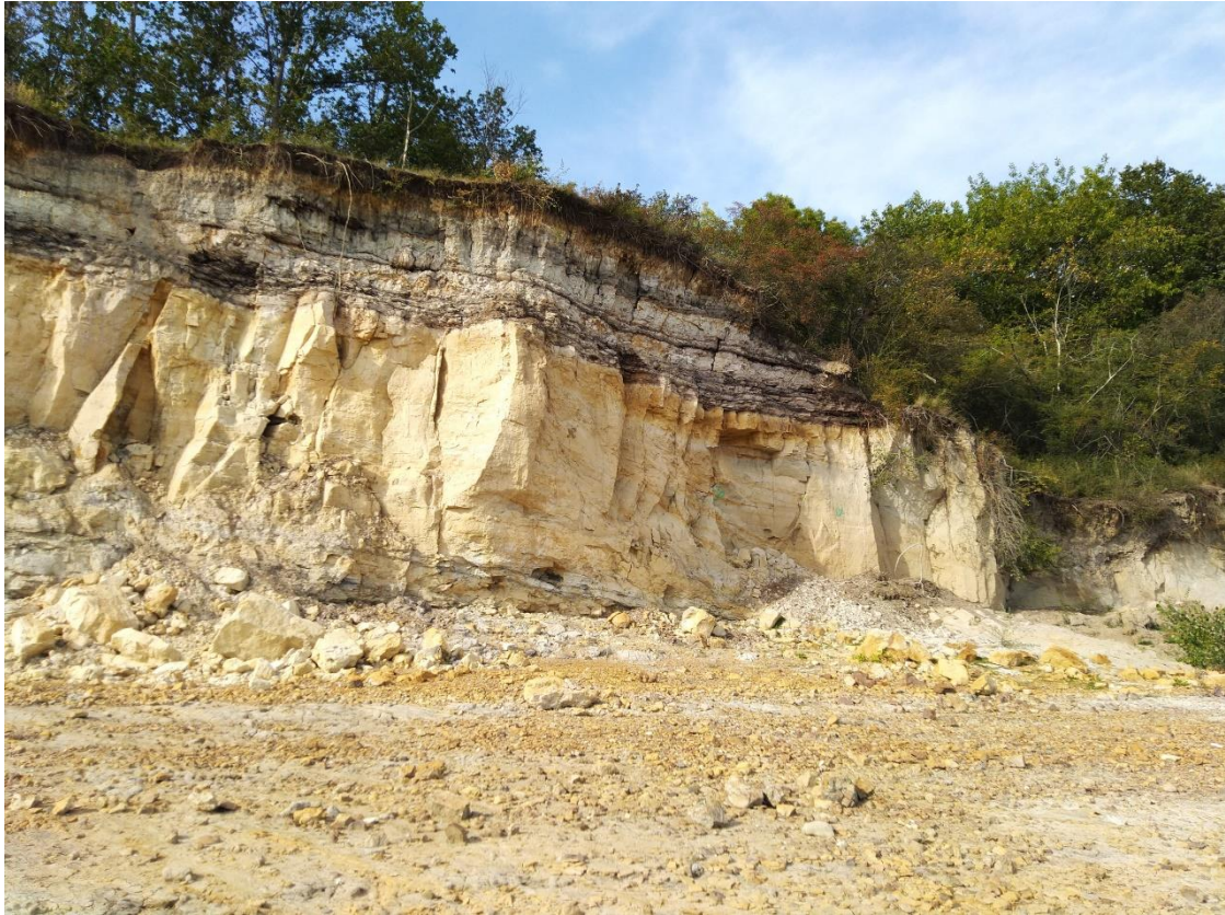
Fig. 18: Nechranice dam: Accumulations of small active rockfalls in clayey and silty sediments
