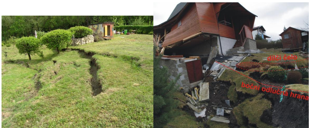
Fig. 12: Poláky: The scarp and damaged house on the Poláky landslide (2014)
