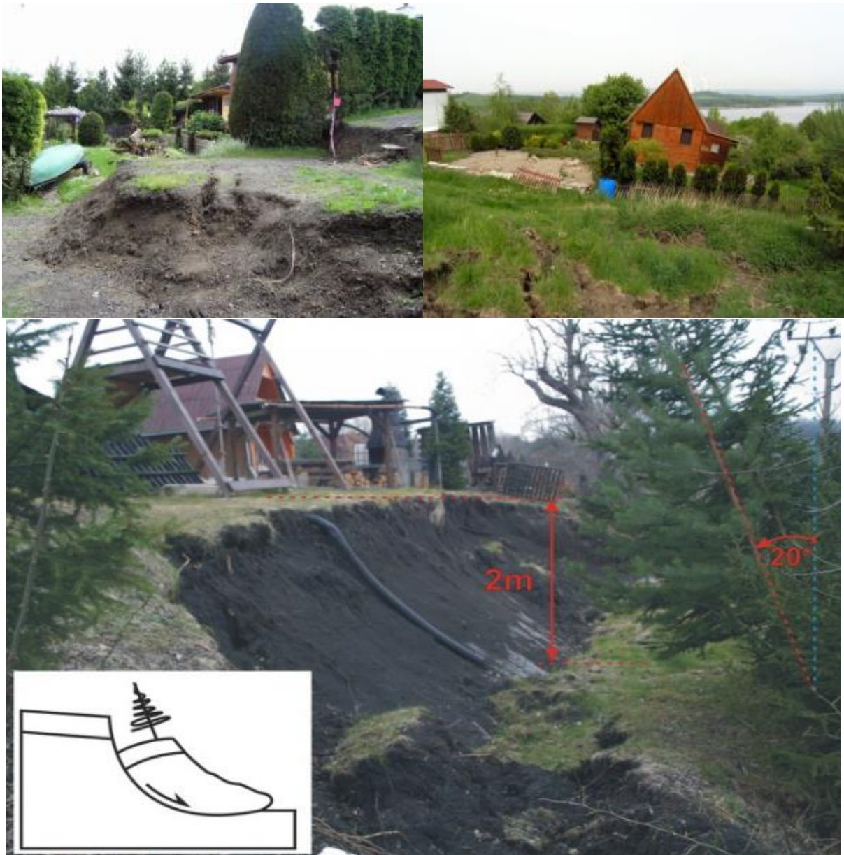
Fig. 11: Poláky: The The scarp and damaged house on the Poláky landslide (2014)
