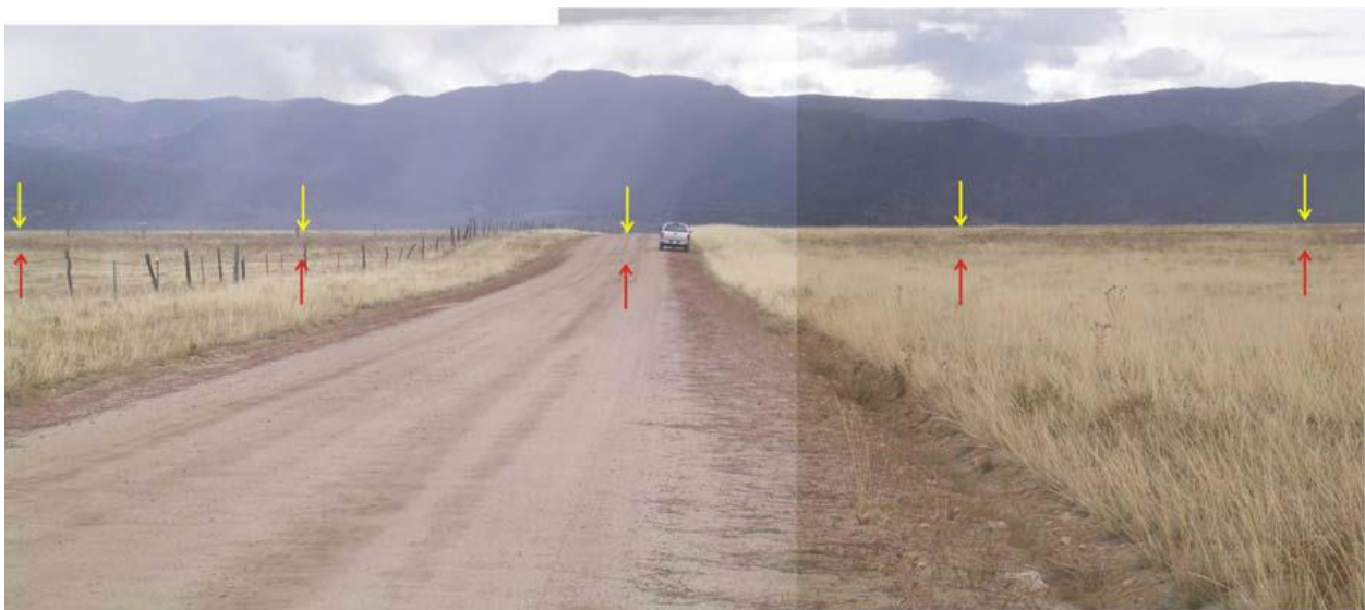
Figure 3-2. View of antithetic fault scarp (between arrows) offsetting Kansan alluvium (Qk) by 2.5-3 m in Maxwell Park. View to east along County Road 328. Pickup truck on scarp is 2.2 m high.
