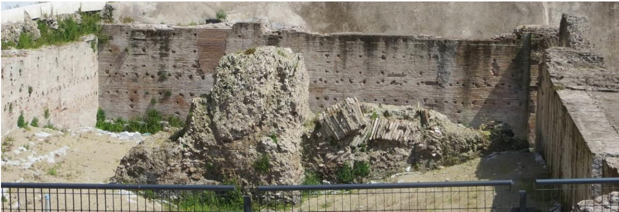
Fig. 2.4.4 – Tumbled down structures of a building of the Hadrian period (Galadini et al., 2013). The tallest block has intruded in a strongly deformed underlying floor.
