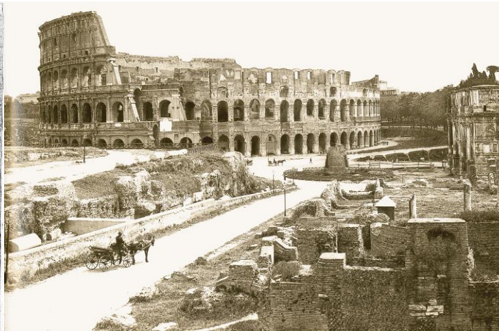
Fig. 2.1.2 - Left (etching of Piranesi, 1776): on the southern side of Colosseum most of the seismically-induced damages occurred. The first two rings are missing and the third one collapsed after the 1703 earthquake. Right: major restorations started only in 1845; they are evident by the smooth red brick surfaces on the travertine. In this Alinari's photograph of the end of 1800, Meta Sudans and Collina Velia (left of the cart) are still present.
