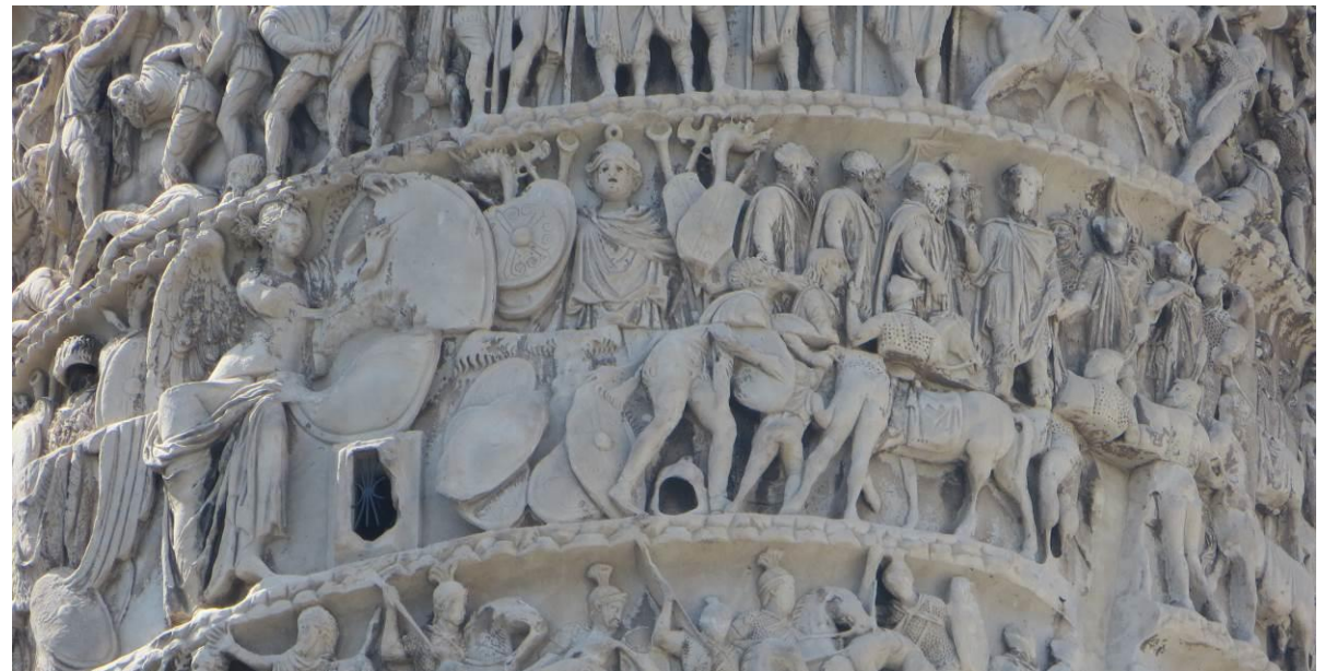
Fig. 2.5.3 – Mismatch of drums between spiral line 9 and 10 from below, side facing the current via del Corso.
